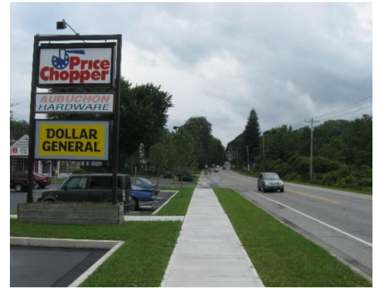
Figure 8: Sidewalk improvements, Windsor
