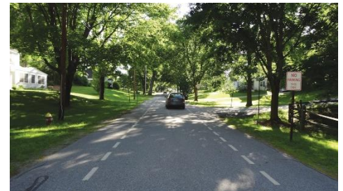
Figure 3: Example of a mixed traffic roadway with advisory shoulders in Hanover.
