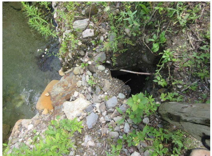
Bottom right: Looking down on destabilized culvert cover. August 2, 2016
