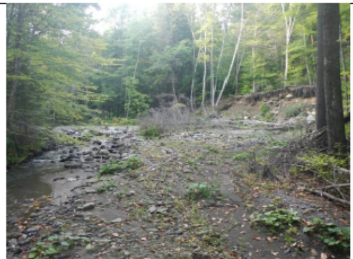
Ongoing widening and erosion/mass failure
