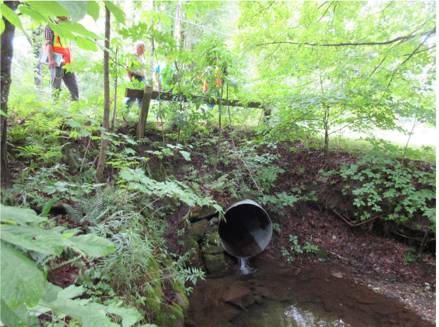
Downstream end of culvert
