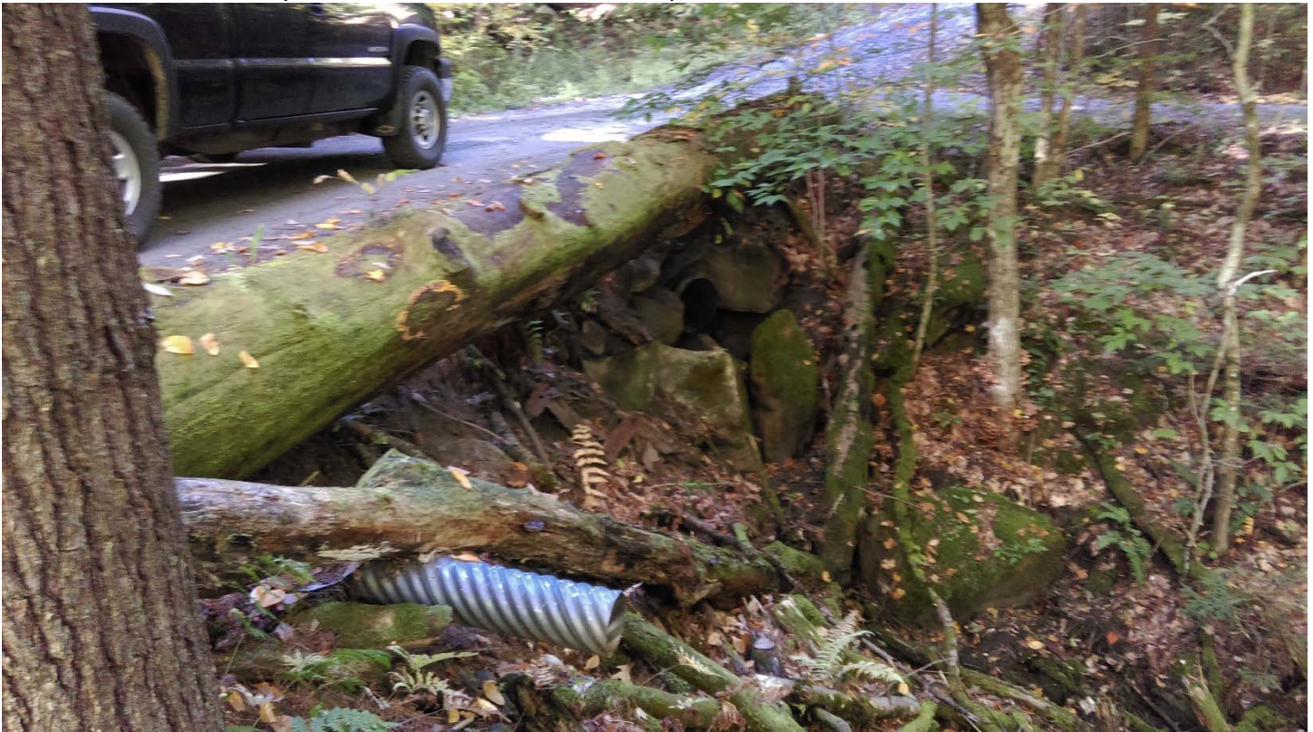
Bottom: Class 4 roadway as seen from the side of the slope.
