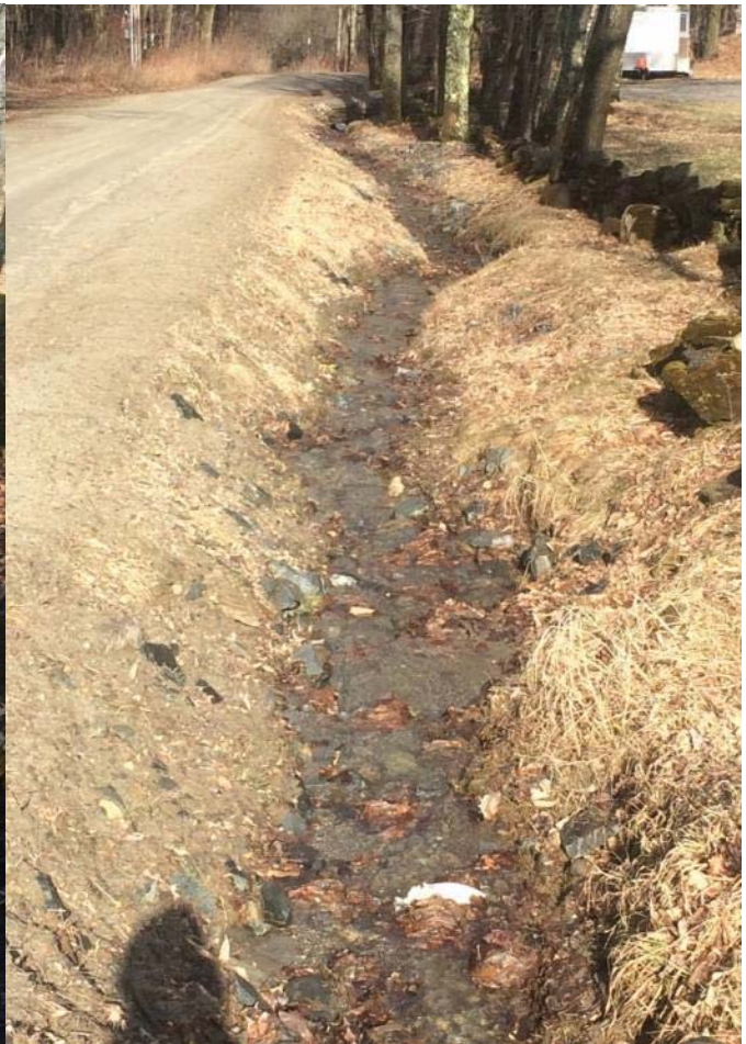
Bottom: Place where ditch turns out to the right into forest. In high water flow water also flows along roadway which turns to the left
