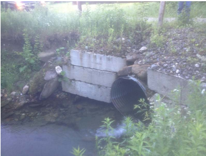
Bottom right: Looking down on destabilized culvert cover. August 2, 2016
