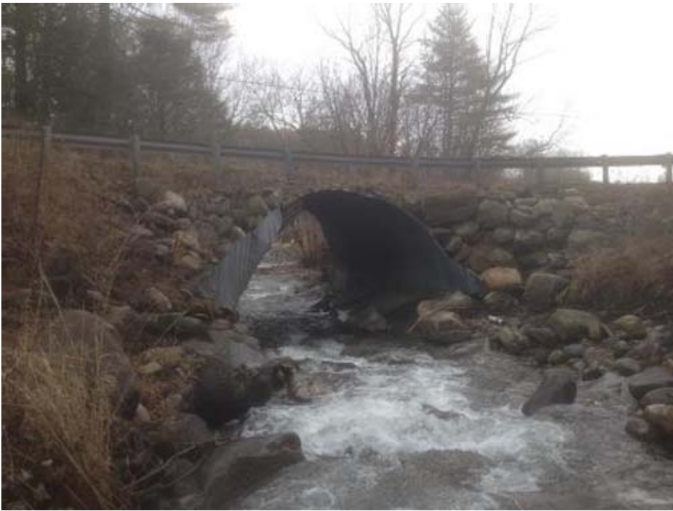
Top: Upstream end of culvert
