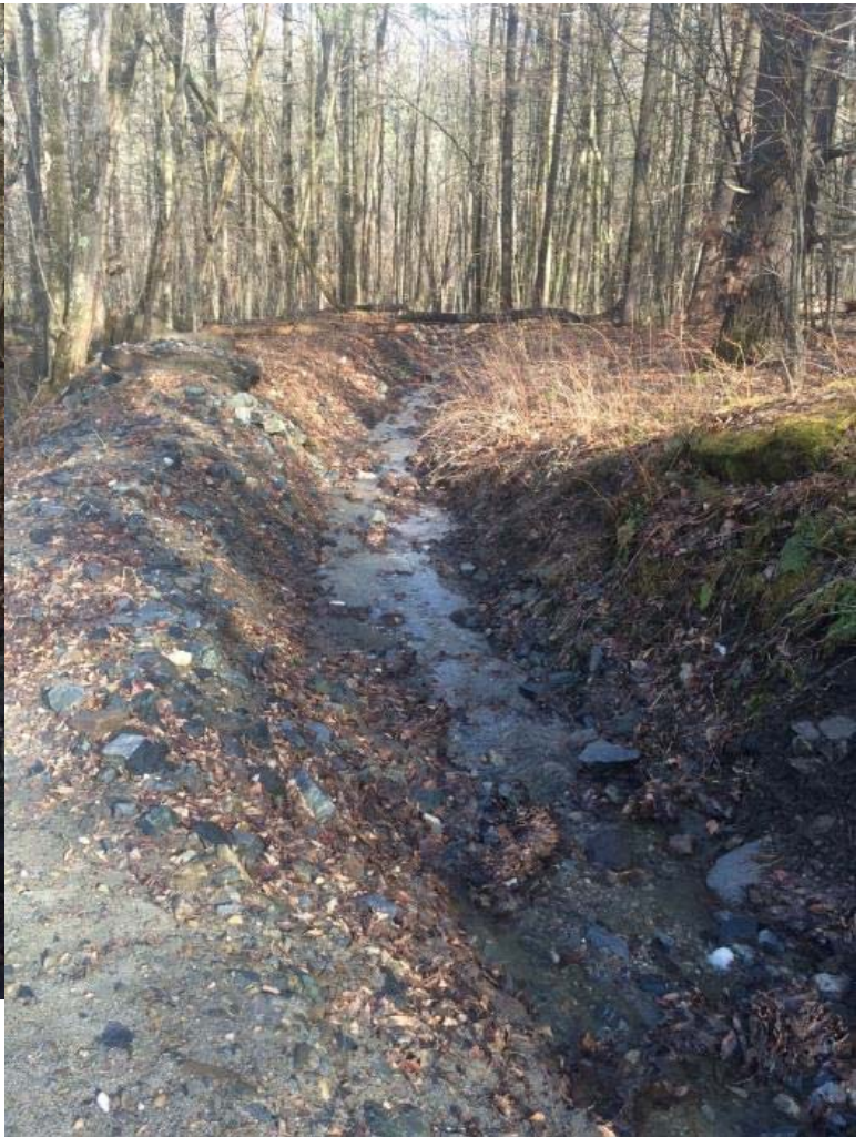
Top Right: Turn out which heads into the woods
