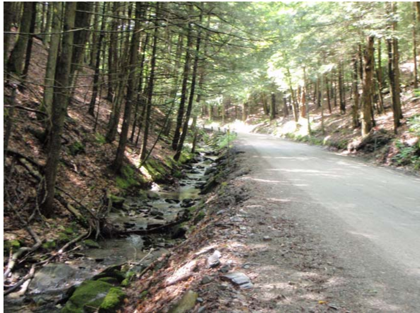
Figure 12. Corridor encroachment along Weeden Hill Road in reach M09
