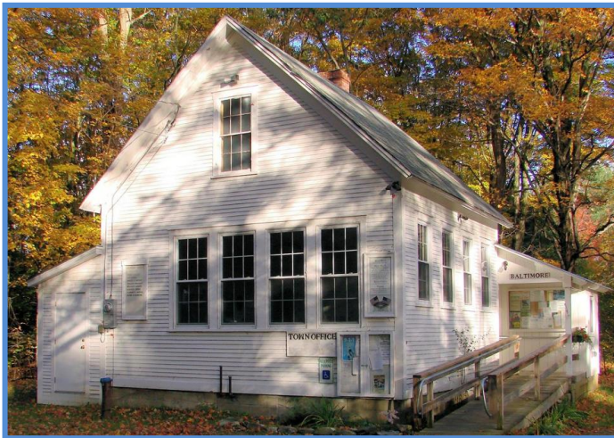
Figure 2: Baltimore's Town Office
