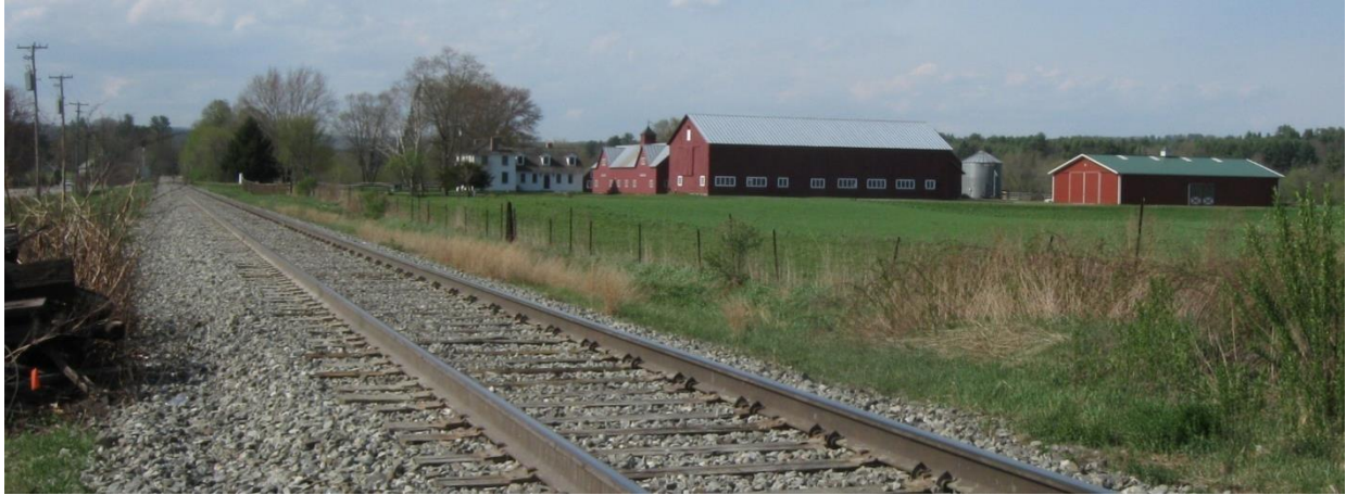
Rail in Windsor.
