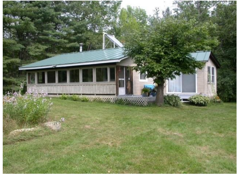
Figure 5: Renewable energy systems were more the exception than the rule in the region in 2015. However, there are a lot more systems being installed in the last few years, such as this solar hot water system (evacuated tubes) on a house in Weathersfield. (Julia Lloyd Wright)
